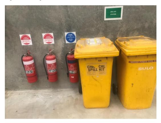
Image 8 – Spill kit and fire extinguishers
